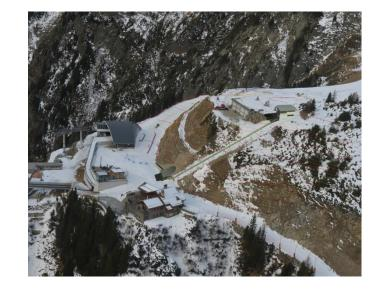
This new lift, called FUNI 2000, operates by the movement of a cabin (of the telecabin type) mounted on a chassis itself moving on rails or tubes. Movement from top to bottom and from bottom to top is achieved by means of a cable which rolls up (when climbing) and unrolls (when descending) from the top station.
